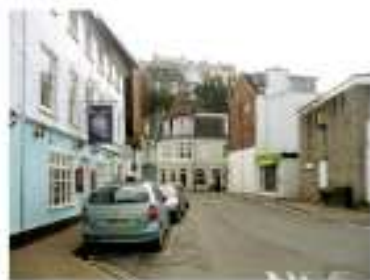
view from Broad Street - existing
